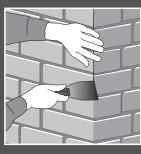
**E.** When the joint is filled, remove any irregularities in the paste with
