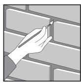
**6.** When filled, remove any irregularities in the paste with a fine brush. Once the paste is completely dry (approx. 24 hours), paint the joints and screw-holes with Panespol special paint, to give a perfect finish.
